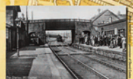
The street scene in Willington, showing the railway station and the street scene.
